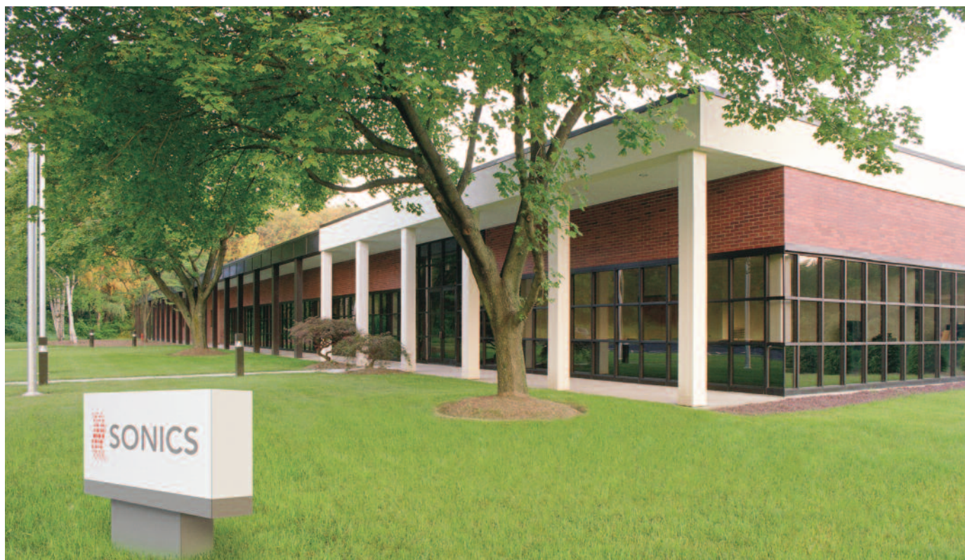
Sonics' worldwide headquarters and manufacturing facility in Newtown, Connecticut, USA
